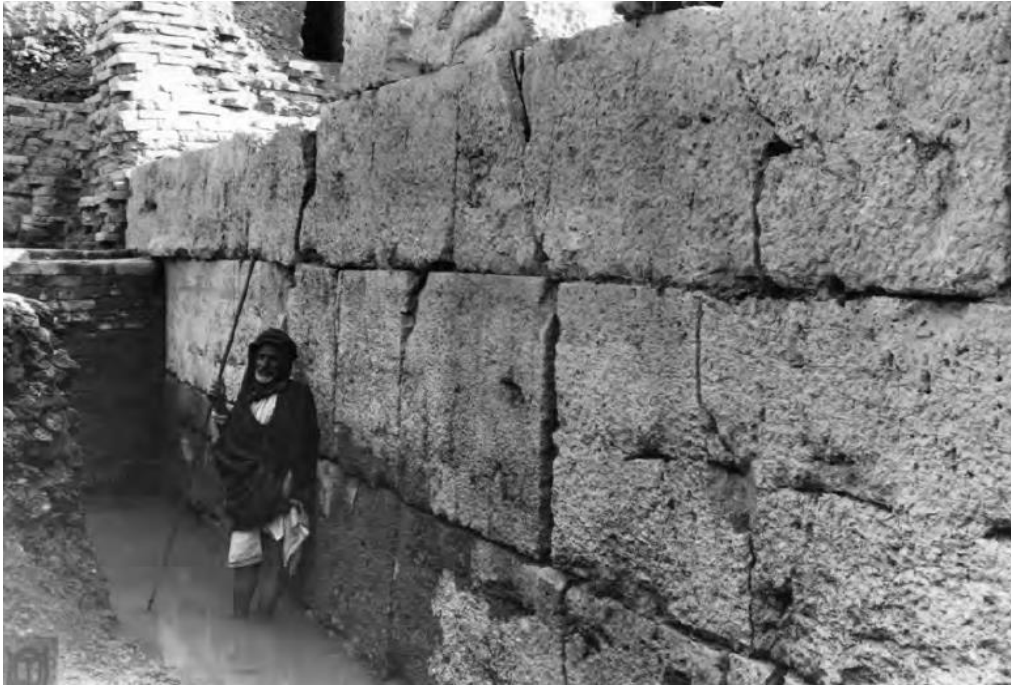
Fig. 1.2. North wall of North Palace with almost one-meter high limestone blocks. Each of the blocks of the middle level has on its upper third, just above the head of the man, a three lines inscription concerning Nebuchadnezzar's construction of the limestone wall of the palace. Top of the stone wall now 2 m under present ground water level. November 1911. PhBab 2508 (DOG, VAM photo archives).
